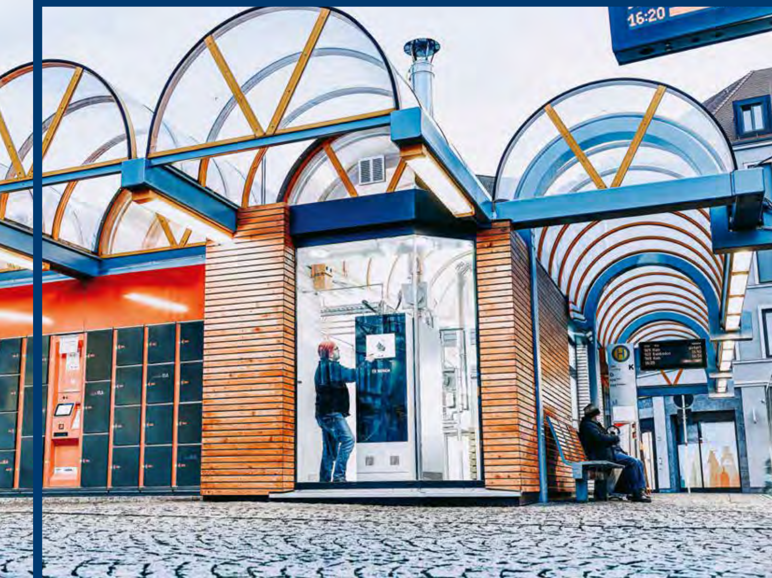
STATIONARY FUEL CELL (SOFC) in the Bamberg omnibus station, Germany
